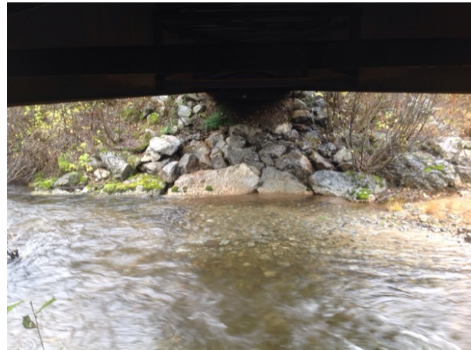
Right Bank Abutment when facing downstream
