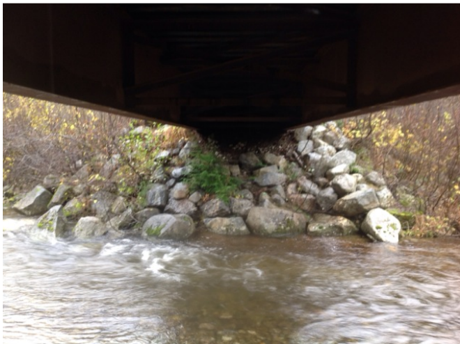
Left Bank Abutment when facing downstream
